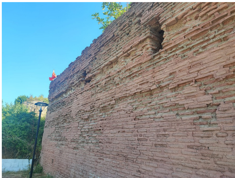
Figure 8: The settlement walls made of bricks.
